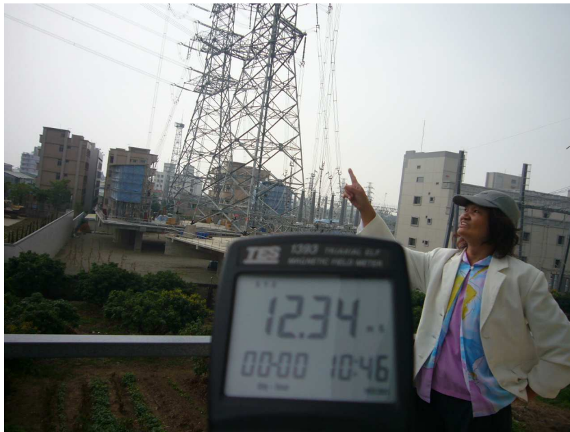
Fig.7 On Zhi-Chiang Street of Wo-Fong Jia-In Village, many high-voltage electricity towers are located close to the community district with many web-like cables carrying this electricity passing over rooftops.
