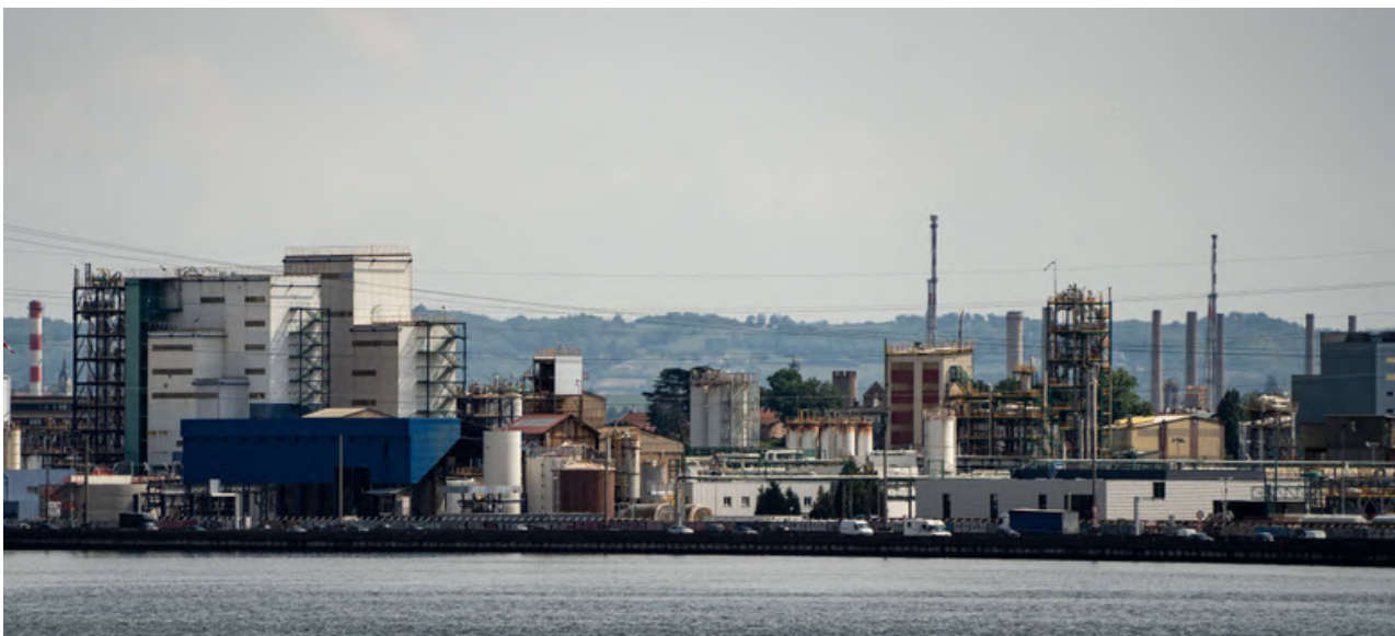
The Arkema plant on the banks of the Rhône, in Pierre-Bénite (France), in May 2022. Credit: Nicolas Liponne/Hans Lucas/AFP.
